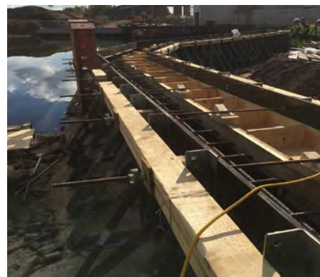
Capping beam with angles and mix of land and river sides
