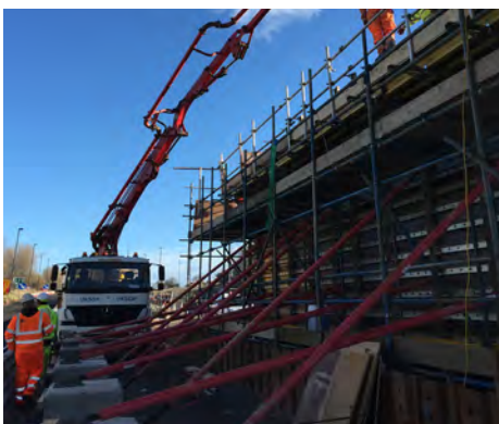
6.4m high motorway central pier with access
