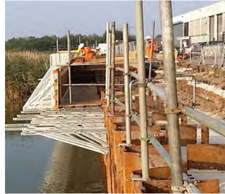
Capping beam with landside formwork
