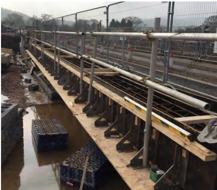
Rail capping beam (3m drop on other side)
