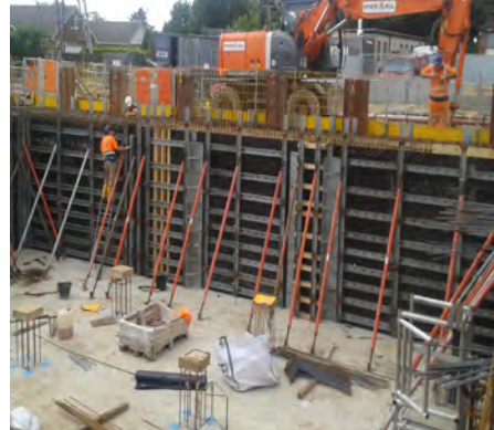
1.9m wall system in use on windfarm control building
