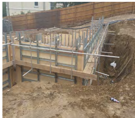
1.9m / 2.4m and 3.2m in use on retaining wing wall
