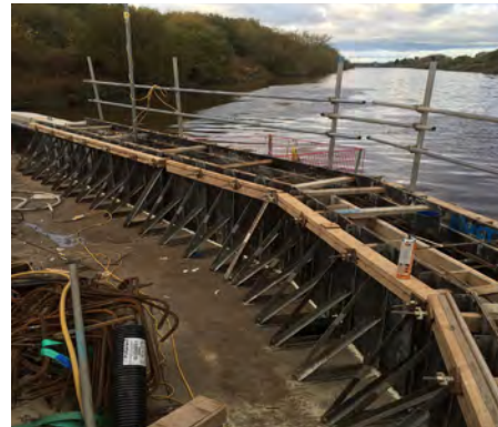
Capping beam with angles and mix of land and river sides
