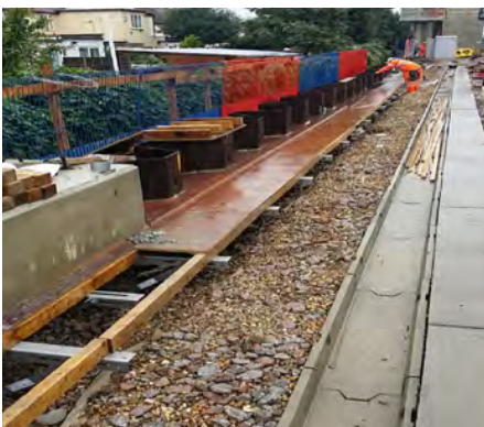
Rail capping beam (3m drop on other side)
