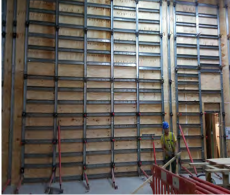
2.4m wall system for cow sheds in Lincolnshire, no props
